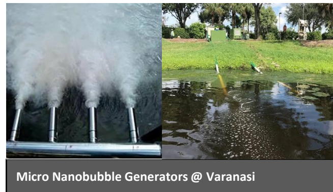
Nanobubble Aerators @ Varanasi
